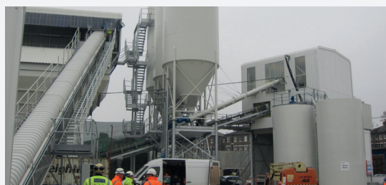
Completed silos with stair access to silo top enclosure.
