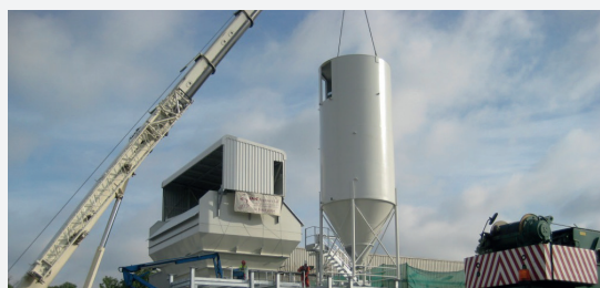
One of the three silos supplied with the new plant being installed on site.
