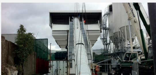
Conveyor being installed on site, by two cranes carrying out a tandem lift.
