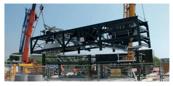
The image below shows the main section of the mortar plant being erected on site.
